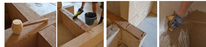
Press the block with a rubber mallet
