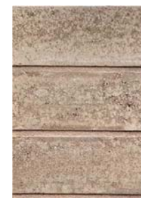
Junta rehundida Raked joint
