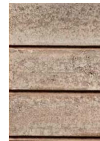
Junta biselada Weathered joint
