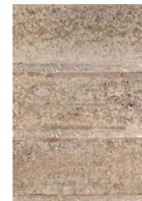
Junta enrasada Flushed joint
