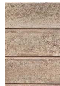
Junta rehundida Raked joint
