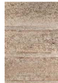
Junta enrasada Flushed joint
