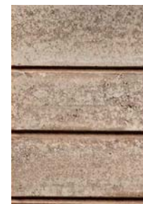
Junta biselada Weathered joint
