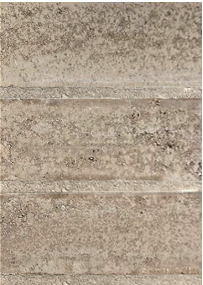
Junta enrasada Flushed joint
