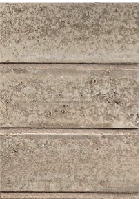
Junta rehundida Raked joint
