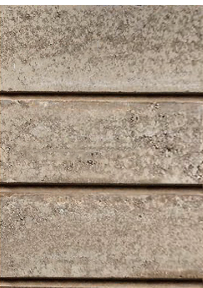
Junta biselada Weathered joint
