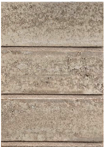
Junta rehundida Raked joint
