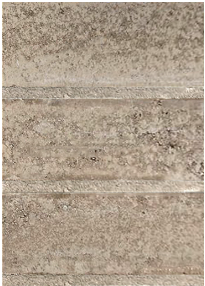
Junta enrasada Flushed joint
